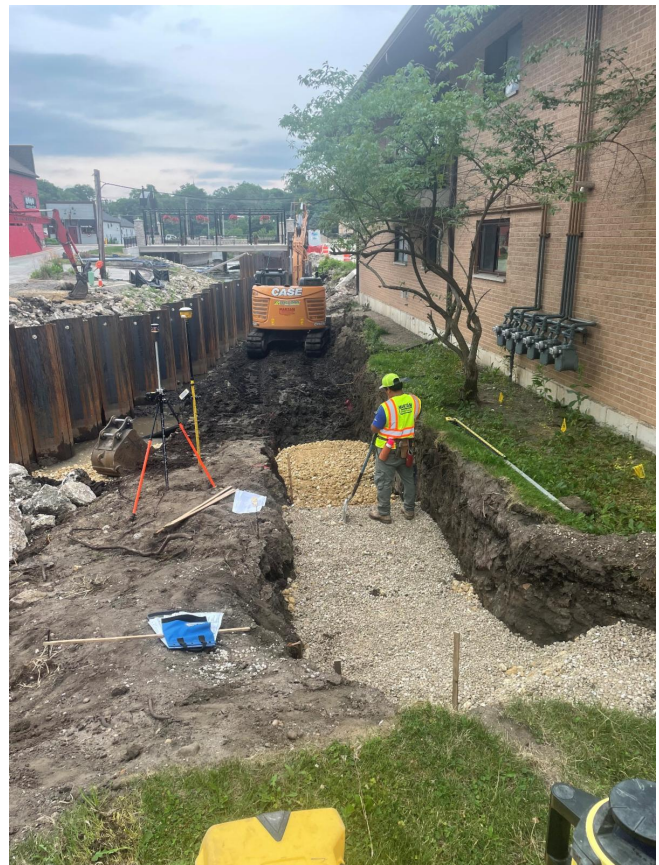
Subbase Placement
