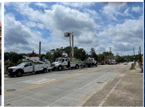
Aerial Utility Work
