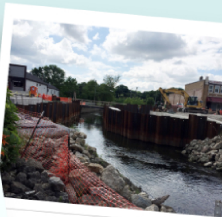
COFFERDAM BUILT AT MAIN STREET
