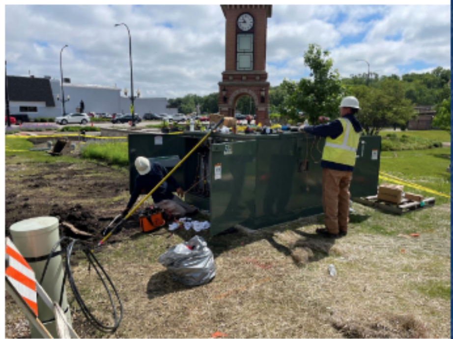
ComEd Switch Gear Installation
