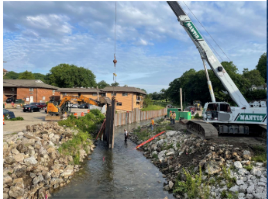
Cofferdam Construction
