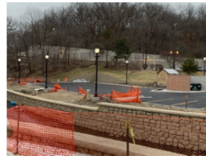
Historic Village Hall Light Pole Installation
