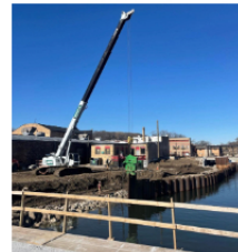
Sheet Pile Removal
