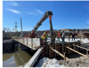
Harrison Street Bridge Abutment
