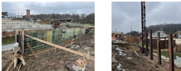
Harrison Street Bridge Abutment Reinforcement Bars and Piles
