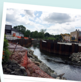
COFFERDAM BUILT AT MAIN STREET
