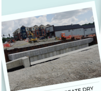
COFFERDAMS CREATE DRY CONSTRUCTION WORK AREAS
