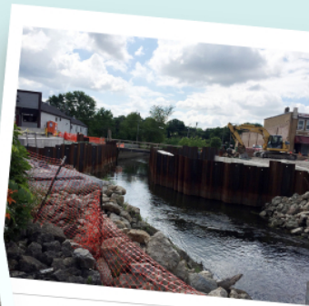
COFFERDAM BUILT AT MAIN STREET
