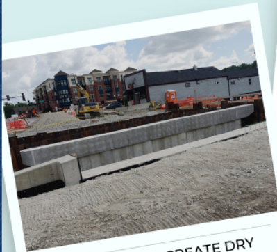
COFFERDAM BUILT AT MAIN STREET
