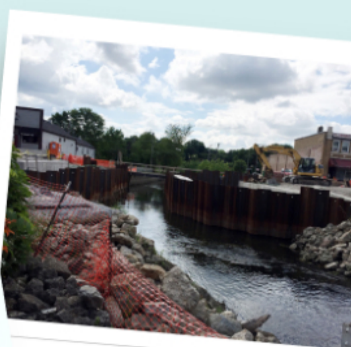
COFFERDAM BUILT AT MAIN STREET
