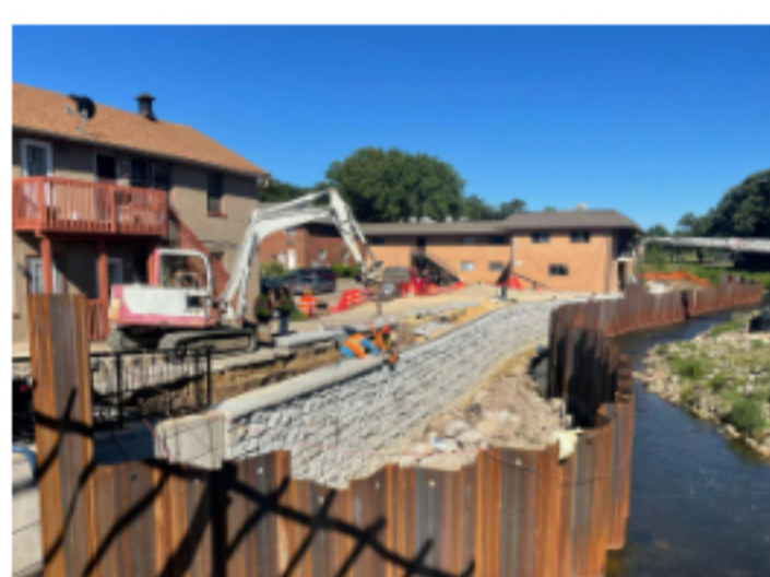
Retaining Wall Construction
