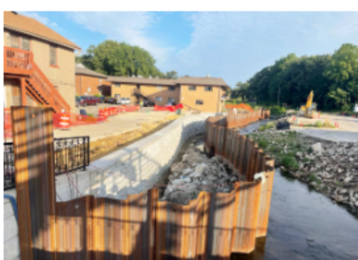
Retaining Wall Completed
