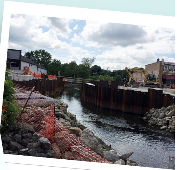
COFFERDAM BUILT AT MAIN STREET
