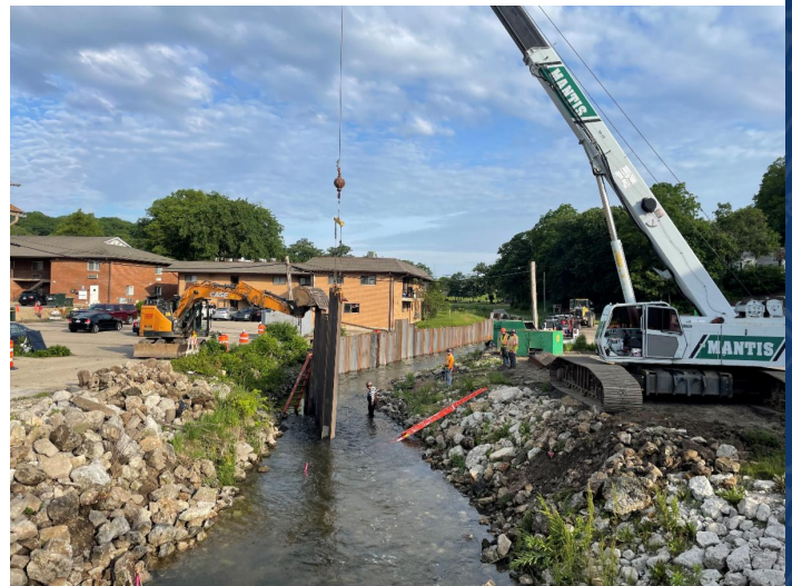
Cofferdam Construction
